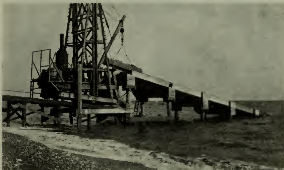
STEPPED GANGWAY PANEL BEING PLACED IN POSITION.
